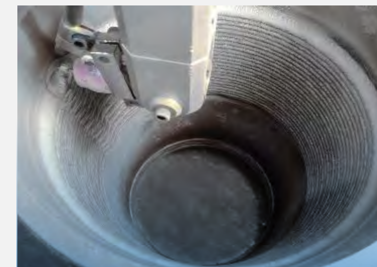
• Auto-TIG Bore Welding
