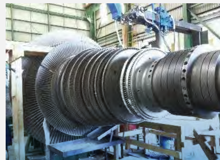
• Sub-Arc Rotor Welding
