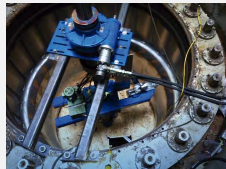
• Boring Bar Setup
