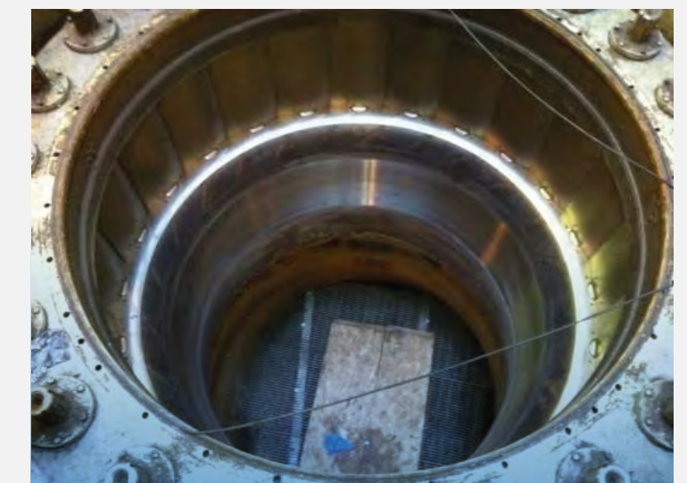
• Bore Restoration Complete
